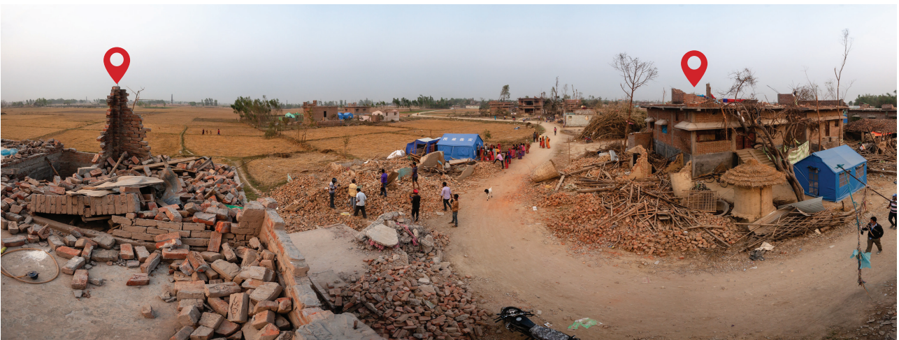
Figure 3.10c: Brick walls of top floor structure collapsed completely in some two-story houses (Pheta)
